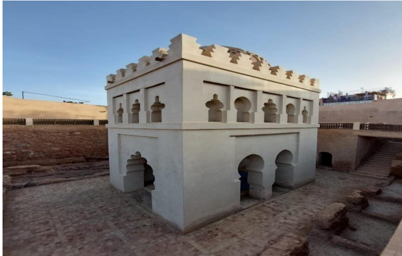
Figure 11: A Recent Photo of Almoravid Dome After Restoration
